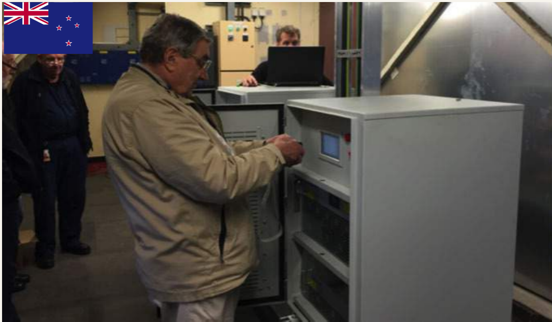
New Zealand, Parliament Library, SVG 200kVar John Fulton was taking photo for SVG performance, because he be surprised at the consistent Cos fi 0.99 by SVG
